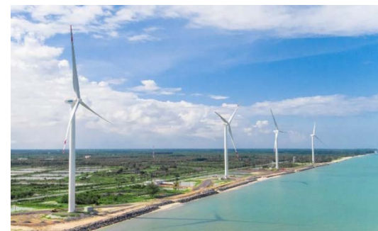
10 MW Wind Power Plant (LLG)
