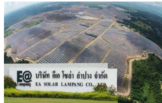
Solar Farm at Lampang, Thailand
