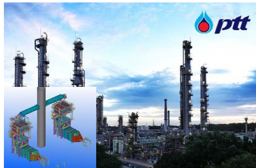
PTT WASTE HEAT RECOVERY SYSTEM FOR GSP NO.5&6 PROJECT
