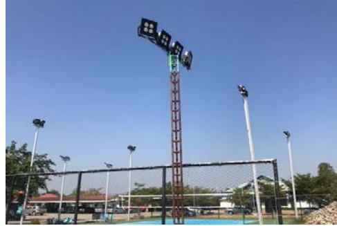
Energy Efficiency Improvement by replace old lighting system to LED at Nong Bua Subdistrict Municipality
