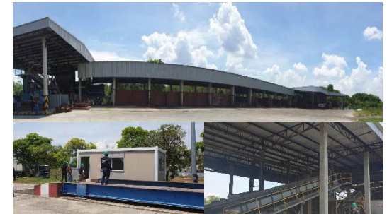
Municipal Solid Waste Management Center of Saraburi Provincial Administrative
