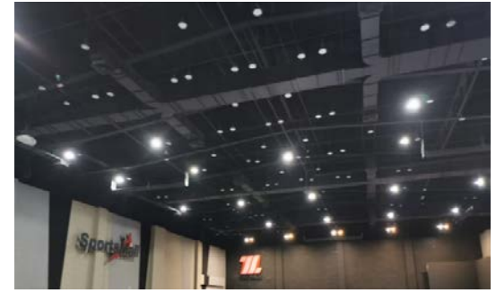
LED Lighting Replacement Project by The Mall Korat
