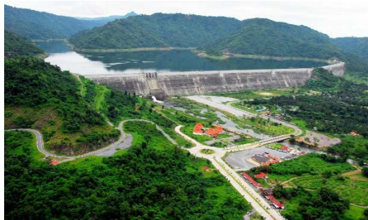
Khun Dan Prakarnchon Hydropower Plant
