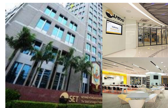
Hi-efficient lighting installation in SET Building
