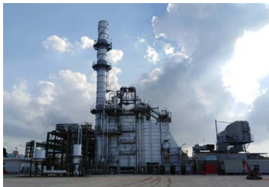
GPSC Cogeneration Plant (Central Utility Plant #4 : CUP-4) Phase 1
