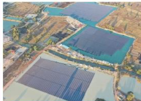
Floating solar power (Thailand) 2,552 tCO 2 /y. Start operation Jan. 2020
