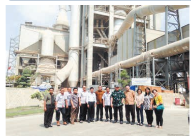
Waste heat recovery in Cement Industry, JFE engineering, Indonesia
