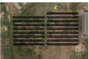
Solar PV System at Salt Factory, PCKK, Kenya
