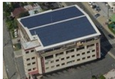
Installing solar PV system, PCKK, Palau Maldives
