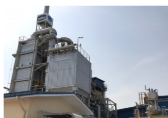
Waste to Energy Plant, JFE engineering, Myanmar
