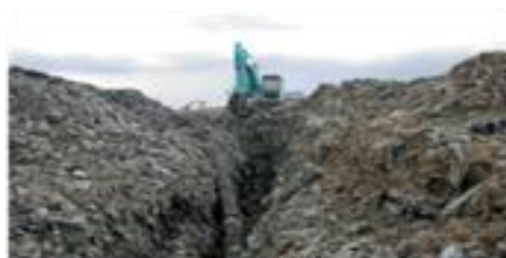
Installation of LFG collection wells
