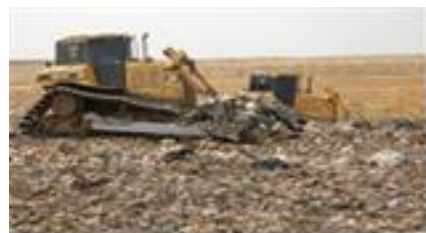
Waste arrives on site
