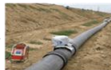
Collected LFG transported via carrier pipes to generation compound
