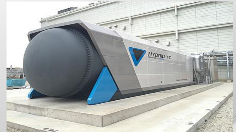
Site Ref. : Fuel Cell-Gas Turbine Hybrid System ของ Mitsubishi Hitachi Power Systems Capacity : 250 Kw
